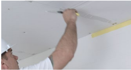
1. Lay the filler on the joints
