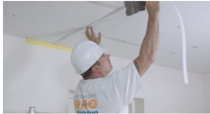
2. While the filler is still wet, position the tape on the joints
